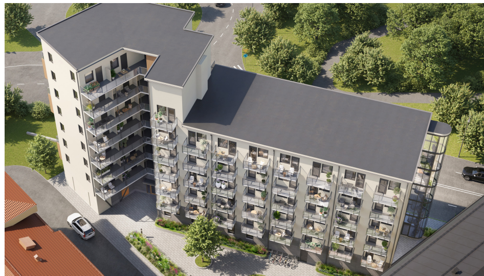
Eddahuset is Klöver's first completed residential building in Uppsala, offering space-efficient one- and two-room apartments, many with balconies. The property is certified according to Miljöbyggnad Silver. Completed and fully leased during the second quarter 2025.
